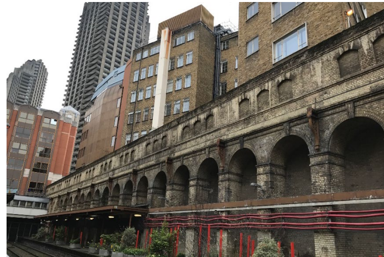
View from Barbican Station platform
